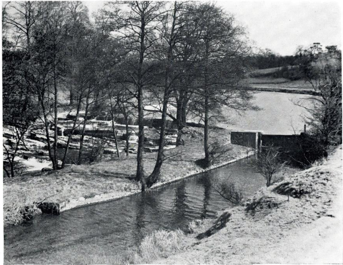
Fig. 7: WEIR ON RIVER RIBBLE AND ENTRANCE TO MILL RACE.
