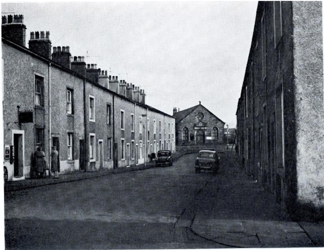
Fig. 16: NELSON STREET, LOOKING EAST.
