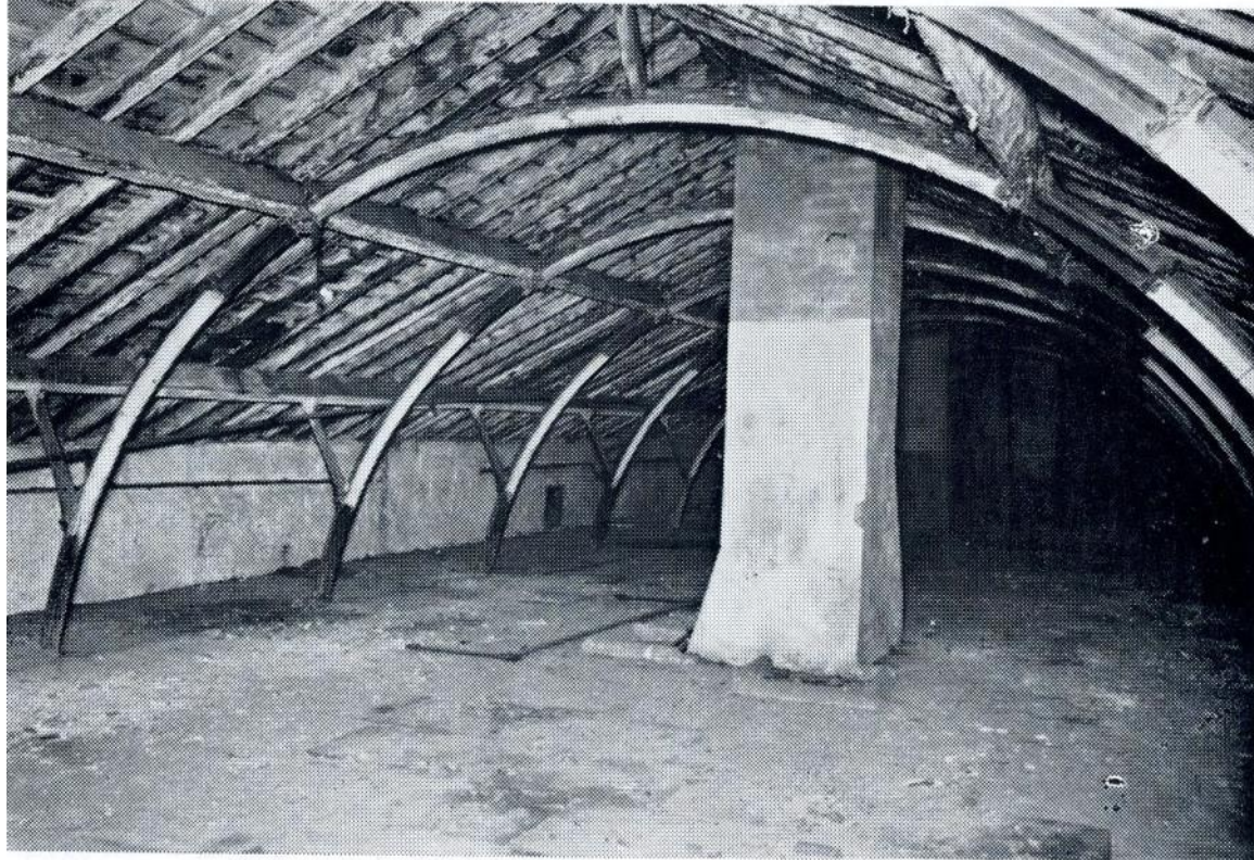
Fig. 12: CAST-IRON ROOF TRUSSES, SOUTH BLOCK.
