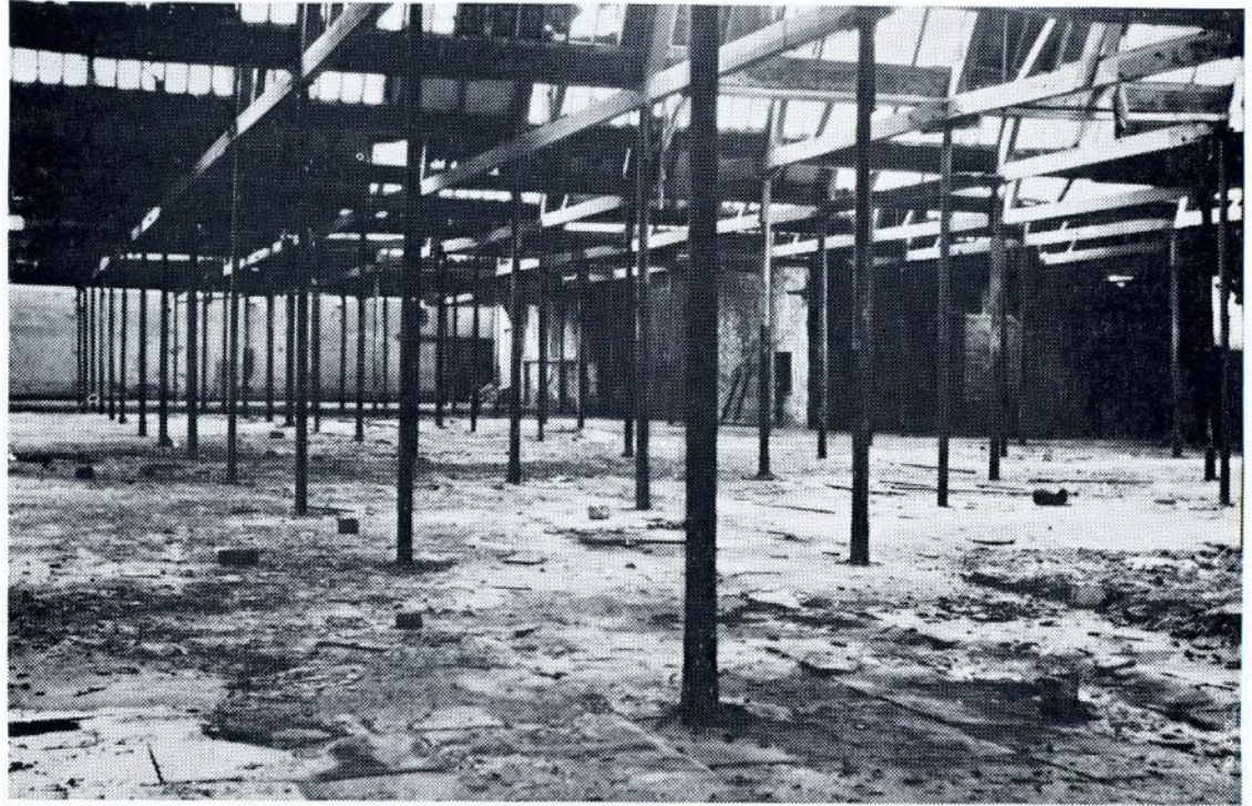
Fig 13: INTERIOR OF WEAVING SHED (new shed).
