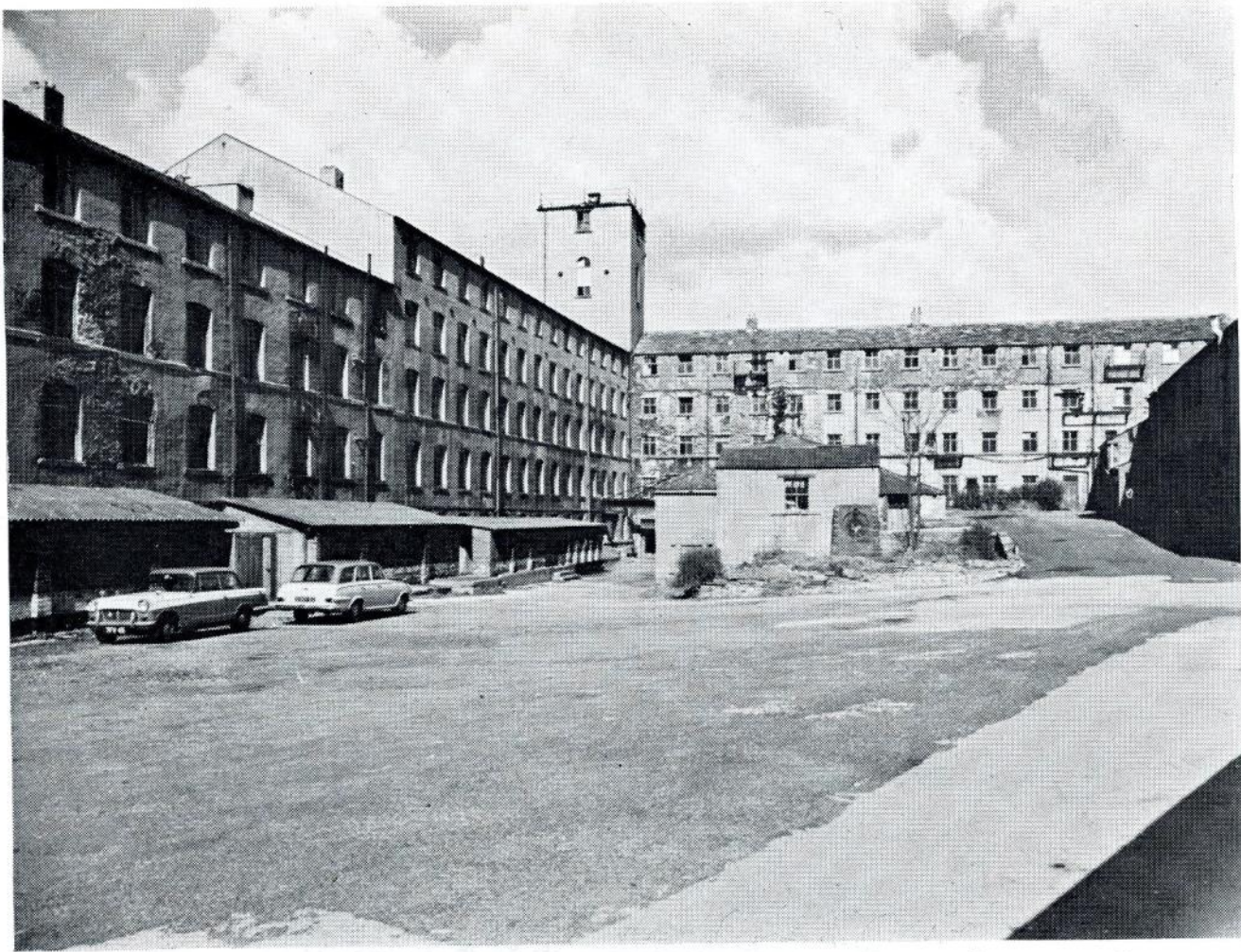
Fig. 6: GENERAL VIEW OF YARD FROM SOUTH-EAST, LOOKING NORTH. SOUTH AND CENTRE SPINNING BLOCKS ON LEFT, EAST BLOCK ON RIGHT.
